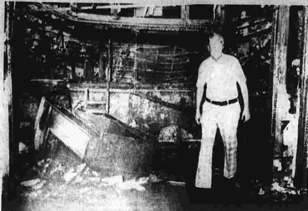
Entrance to burned out night club
